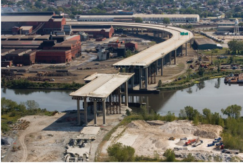
A dismantled portion of the ramp leading to the Cline Avenue Bridge is shown over the Indiana Harbor and Ship Canal in East Chicago in September 2012. (Jon L. Hendricks, The Times)
